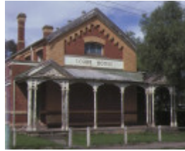
1 wycheproof court house front elevation sep1984
