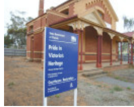
WYCHEPROOF COURT HOUSE SOHE 2008
