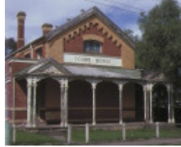
1 wycheproof court house front elevation sep1984
