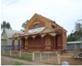
WYCHEPROOF COURT HOUSE SOHE 2008
