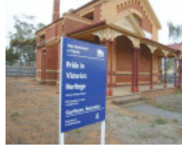
WYCHEPROOF COURT HOUSE SOHE 2008
