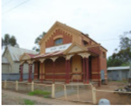
WYCHEPROOF COURT HOUSE SOHE 2008
