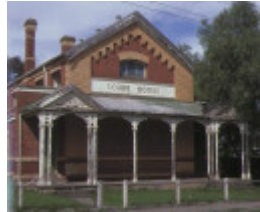
1 wycheproof court house front elevation sep1984
