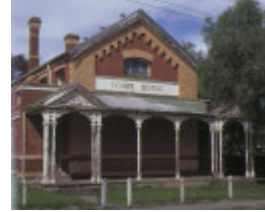
1 wycheproof court house front elevation sep1984
