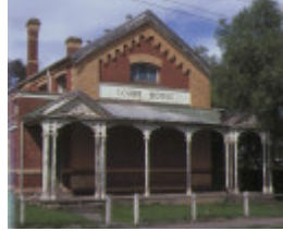
1 wycheproof court house front elevation sep1984
