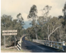
B6396 Bourke's Bridge
