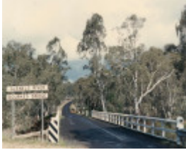
B6396 Bourke's Bridge
