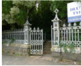
KYNETON ARTS CENTRE (FORMER CONGREGATIONAL CHURCH AND SUNDAY SCHOOL) SOHE 2008
