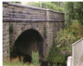
1 bridge over commissioners creek yackandandah side view
