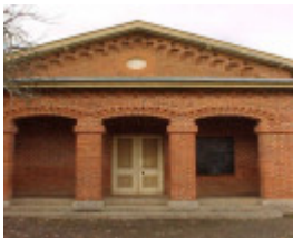
h01490 yackandandah court house 2 pm1 jun03
