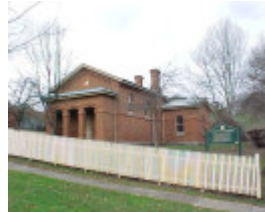
h01490 1 yackandandah court house pm1 jun03
