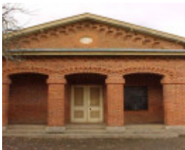
h01490 yackandandah court house 2 pm1 jun03
