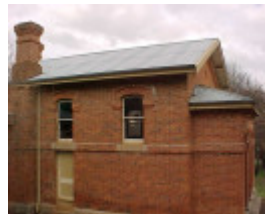
h01490 yackandandah court house 3 pm1 jun03
