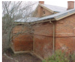
h01490 yackandandah court house 4 pm1 jun03
