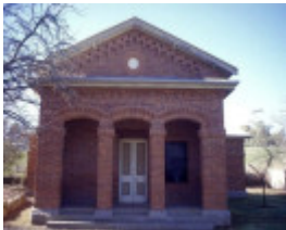
h01490 yackandandah court house williams rd yackandandah porch front she project 2003
