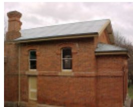
h01490 yackandandah court house 3 pm1 jun03
