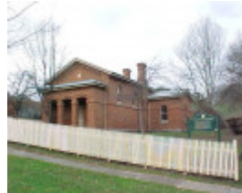
h01490 1 yackandandah court house pm1 jun03
