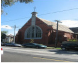
124816 Presbyterian Church Malvern south elevation 2010
