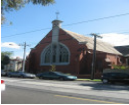
124816 Presbyterian Church Malvern south elevation 2010
