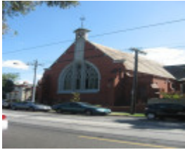
124816 Presbyterian Church Malvern south elevation 2010
