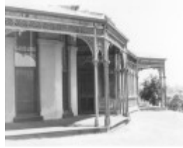
B1207 Clovelly North side looking west.jpg
