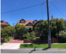
22 Allenby Avenue, Malvern East
