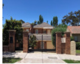
23 23a Allenby Avenue, Malvern East
