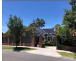
29 Allenby Avenue, Malvern East
