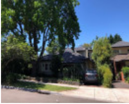
33 Allenby Avenue, Malvern East
