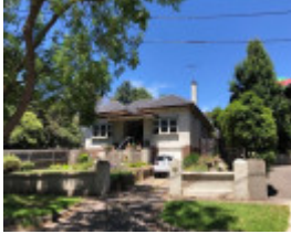
39 Allenby Avenue, Malvern East
