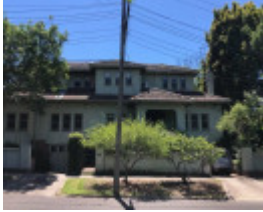
1 Stanley Street, Malvern East
