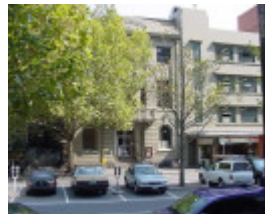
h02001 former victoria carpark
