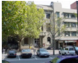
h02001 former victoria carpark
