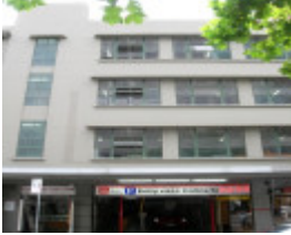
FORMER VICTORIA CAR PARK SOHE 2008
