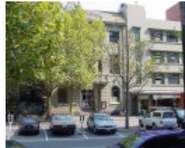
h02001 former victoria carpark
