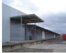
HO189(2) - Former Tottenham Bulk Stores, Beachley Street, Braybrook.JPG
