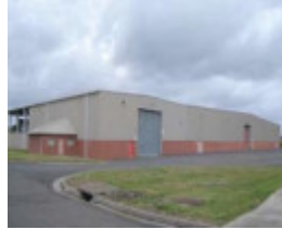
HO189(3) - Former Tottenham Bulk Stores, Beachley Street, Braybrook.JPG
