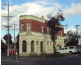
Edwardian commercial building, 68-70 Armadale Street
