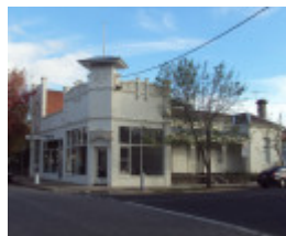
Late Edwardian shops and attached Victorian residence on the corner of Armadale Street and Fetherston Street
