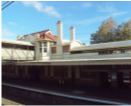
Armadale Railway Station
