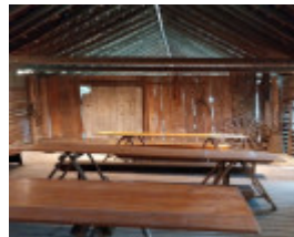
Shingle ceiling in the shed, 2023.
