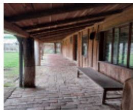
verandah to kitchen block, 2023.
