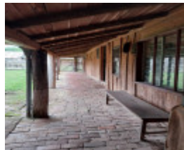
verandah to kitchen block, 2023.
