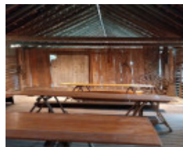
Shingle ceiling in the shed, 2023.
