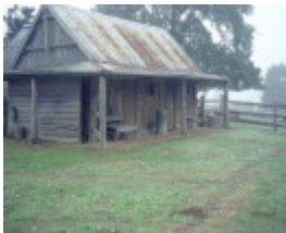
h00384 1 gulf station melba hwy yarraglen butchers shop she project 2003
