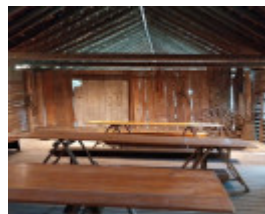
Shingle ceiling in the shed, 2023.
