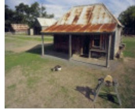
h00384 gulf station melba hwy yarraglen school room she project 2003
