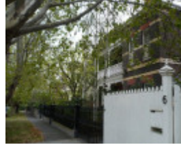
SORRETT AVE LOOKING EAST
