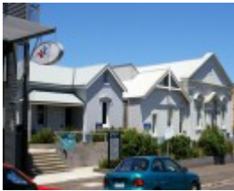
H543 orderly room residence kepler st1
