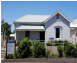
H543 orderly room residence
