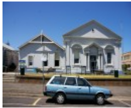
H543 orderly room gun room
