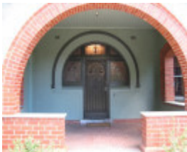
23 Mitford St - entrance porch
