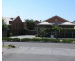
FORMER ROYAL AUSTRALIAN FIELD ARTILLERY BARRACKS SOHE 2008
