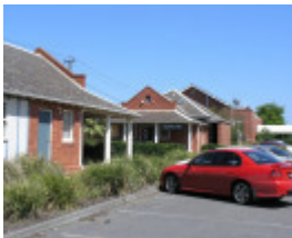
FORMER ROYAL AUSTRALIAN FIELD ARTILLERY BARRACKS SOHE 2008
