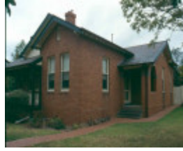
h01098 rafa barracks captain s quarters 2002
