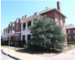
FORMER ROYAL AUSTRALIAN FIELD ARTILLERY BARRACKS SOHE 2008
