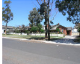
FORMER ROYAL AUSTRALIAN FIELD ARTILLERY BARRACKS SOHE 2008
