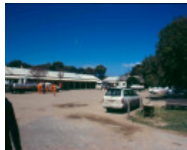
h01090 fort franklin portsea barracks and parade ground 0903 mz
