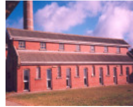
H02030 point nepean bathhouse2
