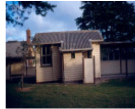
H02030 point nepean isolation hospital
