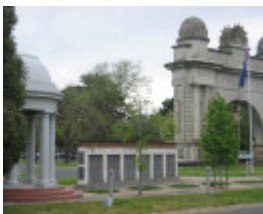
PROV2089 Avenue of Honour Arch Victory 10.05 Precint
