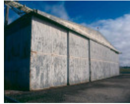
H01969 pt cook bellman hangar aug02 pm1
