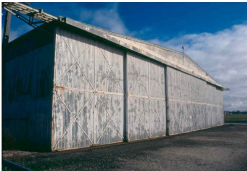
H01969 pt cook bellman hangar aug02 pm1
