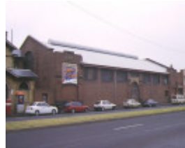
1 naval drill hall side view oct1997
