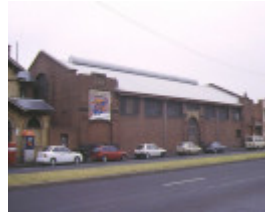
1 naval drill hall side view oct1997
