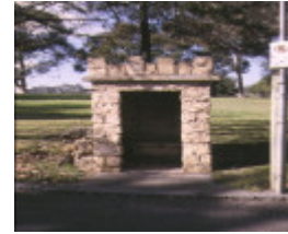
ANZAC Hall Brens Drive Royal Park Parkville Drive
