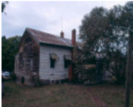
H02024 prefab house maroondah hway rear
