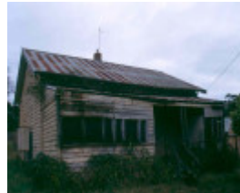
H02024 1 prefab house maroondah hway
