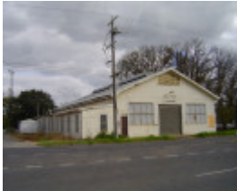
6168 Warragul Drill hall may07 ac 4
