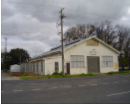
6168 Warragul Drill hall may07 ac 4
