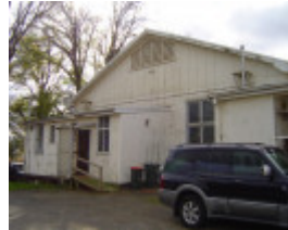
6168 Warragul Drill hall may07 ac 10
