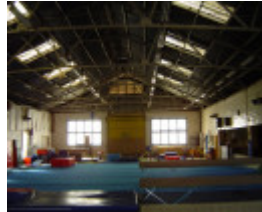
6168 Warragul Drill hall may07 ac 16
