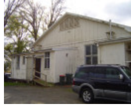
6168 Warragul Drill hall may07 ac 10
