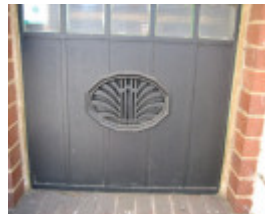
11488 Royal Melbourne Regiment Drill Hall Vent Detail 11 Sept 2006 mz
