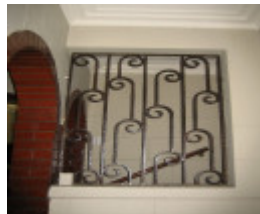
11488 Royal Melbourne Regiment Drill Hall Wrought Iron Screen Detail 11 Sept 2006 mz
