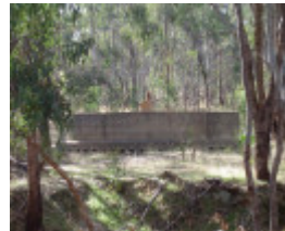
14271 Seymour Light Horse Park May 06 filtration system
