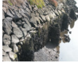
Jack's Magazine Canal And Wharf Maribyrnong July 2003 002
