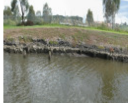
Jack's Magazine Canal And Wharf Maribyrnong July 2003 003
