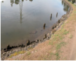
Jack's Magazine Canal And Wharf Maribyrnong July 2003 001
