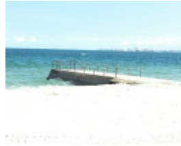
Harold St Drain Port Melbourne April 2006 002
