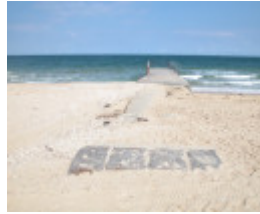
Harold St Drain Port Melbourne April 2006 003
