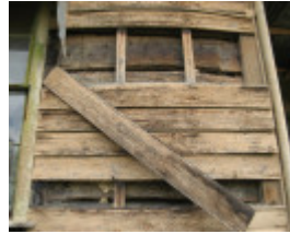
Castlemaine military quarters_slabs under weatherboards_KJ_7 Feb 08
