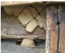
Fmr Castlemaine military quarters_slabs and plaster_Kj_7 Feb 08
