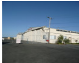
FORMER BALLARAT RAAF BASE SOHE 2008
