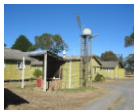
14247 Former Ballarat RAAF Base
