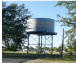
FORMER BALLARAT RAAF BASE SOHE 2008
