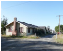
FORMER BALLARAT RAAF BASE SOHE 2008
