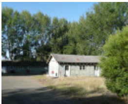
FORMER BALLARAT RAAF BASE SOHE 2008
