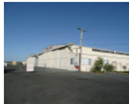
FORMER BALLARAT RAAF BASE SOHE 2008
