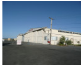
FORMER BALLARAT RAAF BASE SOHE 2008
