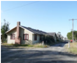
FORMER BALLARAT RAAF BASE SOHE 2008
