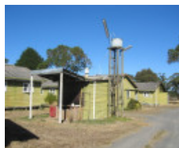
14247 Former Ballarat RAAF Base
