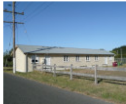
FORMER BALLARAT RAAF BASE SOHE 2008
