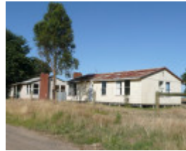
FORMER BALLARAT RAAF BASE SOHE 2008
