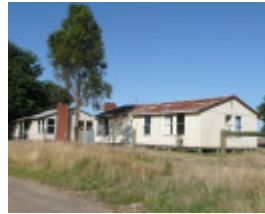
FORMER BALLARAT RAAF BASE SOHE 2008
