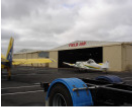
14247 Former Ballarat RAAF base Bellman Hangars
