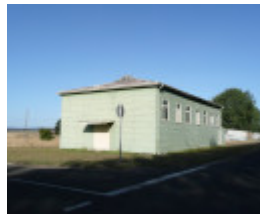
FORMER BALLARAT RAAF BASE SOHE 2008
