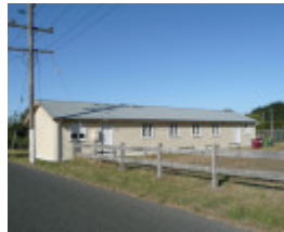
FORMER BALLARAT RAAF BASE SOHE 2008
