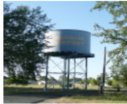
FORMER BALLARAT RAAF BASE SOHE 2008
