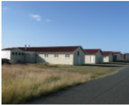
FORMER BALLARAT RAAF BASE SOHE 2008
