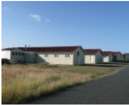
FORMER BALLARAT RAAF BASE SOHE 2008
