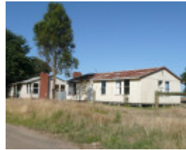
FORMER BALLARAT RAAF BASE SOHE 2008
