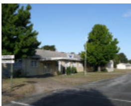
FORMER BALLARAT RAAF BASE SOHE 2008
