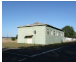
FORMER BALLARAT RAAF BASE SOHE 2008
