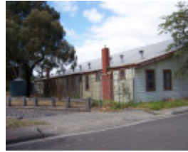
14383 Dandenong drill hall 26oct06 28
