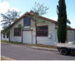
14383 Dandenong drill hall 26oct06 26
