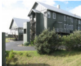
Barwon_Heads_Golf_Club_June_2010 new wings at rear.jpg
