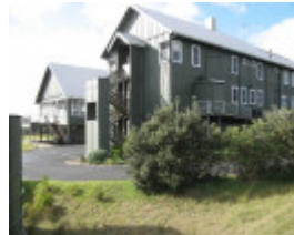
Barwon_Heads_Golf_Club_Jur new wings at rear.jpg
