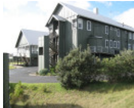
Barwon_Heads_Golf_Club_Jur new wings at rear.jpg
