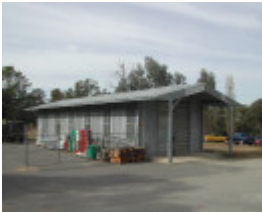
Building Trades Store (No. 029), from the north west
