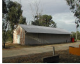
Store S386 from the west
