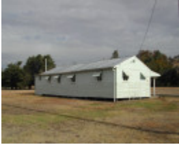
Field Training Storehouse, from the north
