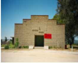
Baranduda Hall, front (west) elevation
