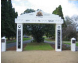
29405 Memorial Arch 1 Walnut Street Whittlesea 25
