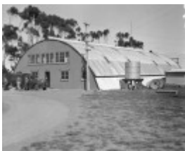
Diggers Rest, 1945. 'Exterior view of the new Igloo Building housing land headquarters signals. (Australian War Memorial)
