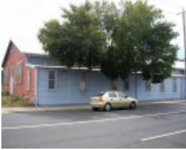
HO93 (1) - Drill Hall, 395 Barkly Street, West Footscray.JPG
