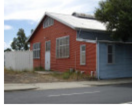
HO93 (2) - Drill Hall, 395 Barkly Street, West Footscray.JPG
