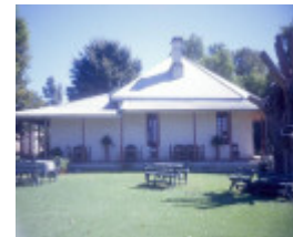
byramine homestead murray valley hwy yarrawonga side of homestead she project 2003
