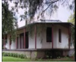
1 byramine homestead front view homestead
