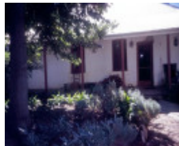
byramine homestead murray valley hwy yarrawonga rear of homestead she project 2003
