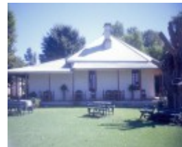
byramine homestead murray valley hwy yarrowonga side of homestead she project 2003
