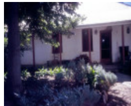
byramine homestead murray valley hwy yarrowonga rear of homestead she project 2003
