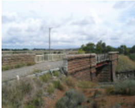
ROAD OVER RAIL BRIDGE SOHE 2008
