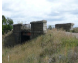
ROAD OVER RAIL BRIDGE SOHE 2008
