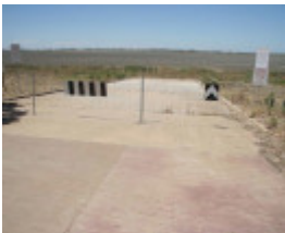
H2208 Boga Slipway Feb 09 PM2
