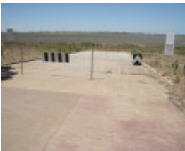
H2208 Boga Slipway Feb 09 PM2
