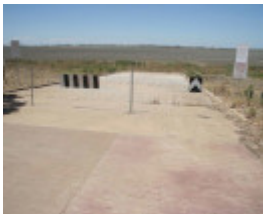
H2208 Boga Slipway Feb 09 PM2
