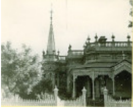
B0592 RSL Sub-Branch 23 Loch St West St Kilda
