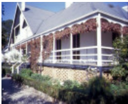
h00371 murrindindi station melba hwy yea homestead east elevation close up she project 2003
