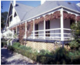
h00371 murrindindi station melba hwy yea homestead east elevation close up she project 2003
