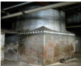
h02067 kinnears ropeworks footscray boiler house chimney base 0703 mz
