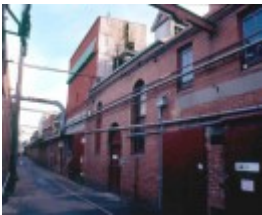
h02067 kinnears ropeworks footscray boiler house external 0703 mz
